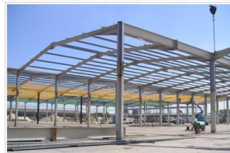
Column splices used to increase the height of the existing building
