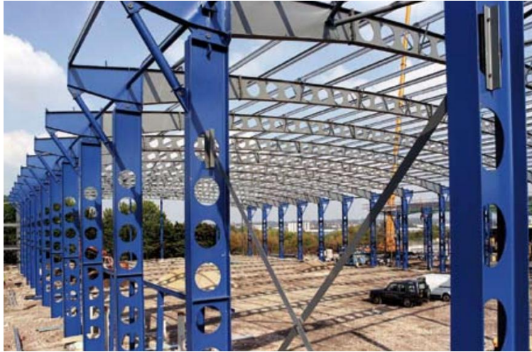
Cellular columns and rafters
