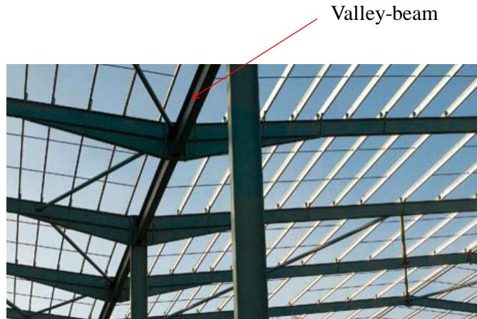
Valley-beam details for “hit” and “miss” frame
