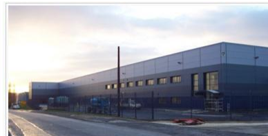
.....and after refurbishment
