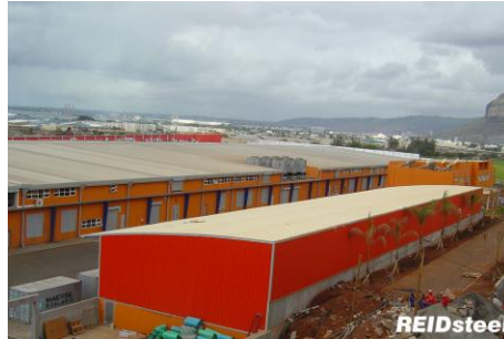
CMT Bale Press Textile Factory Size: 24m x 80m with its curved roof, eave overhang and rounded gutter
